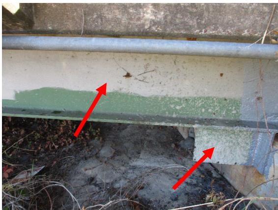
Photo 5. LBP on Gray Steel Girders and Green Steel Girder Brackets.
