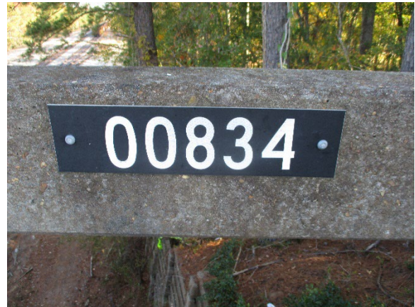
Photo 2. Bridge Asset Number Mounted to Concrete Guardrail.
