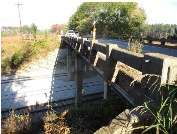
Photo 3. Southwest Corner View of Bridge.
