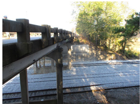
Photo 4. Southeast Corner View of Bridge.
