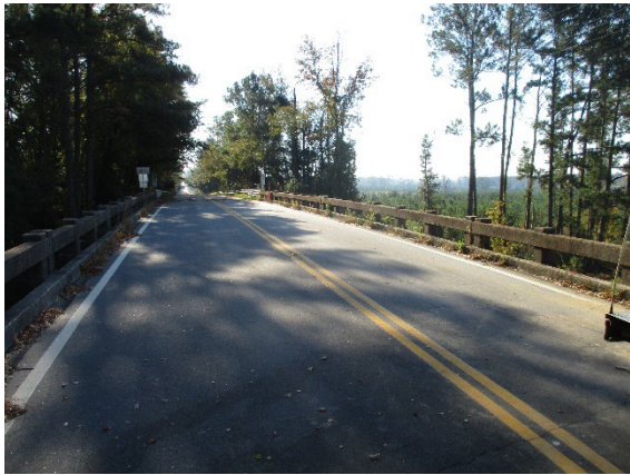
Photo 1. Top View of Bridge.
